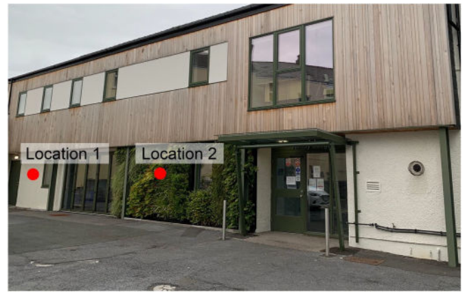
Fig. 3. Photo of case study building, showing locations of monitoring setup.
